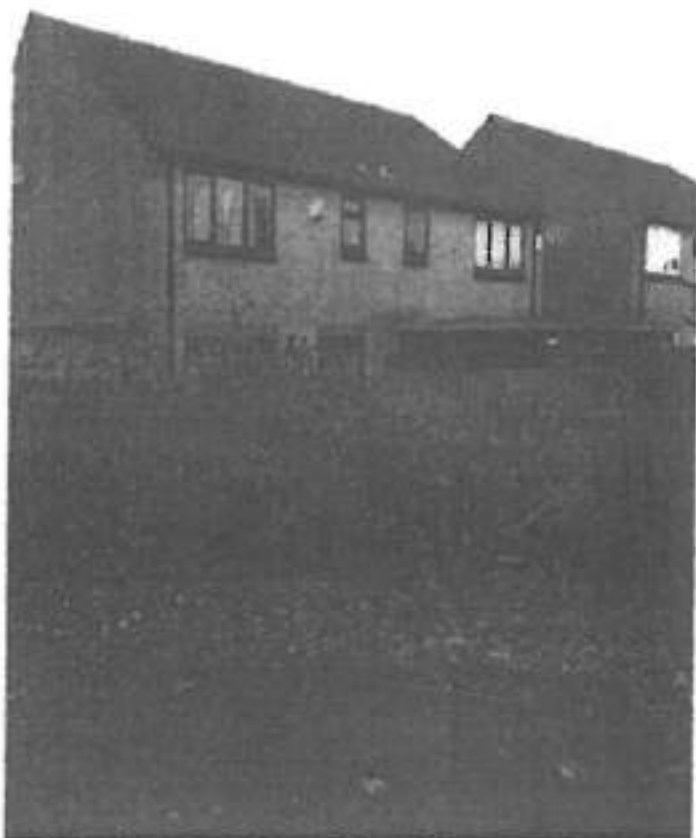
View from behind property when walking along Alkerden Lane. Number 10 to right hand side with conservatory on lower level.
