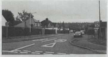
calming measures may be needed to go along with the introduction of the change in the speed limit. This can include gateway treatments, speed humps, chicanes, road narrowing, and other measures to both physically and visually reinforce the reduced speed limit.
